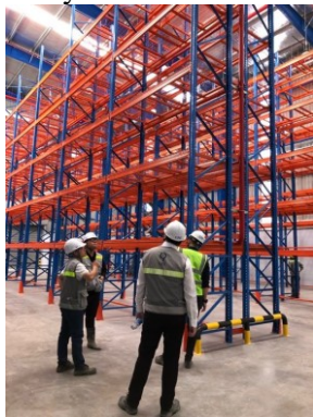
Fig. 1 Akazo Nobel-Material Storage Room
