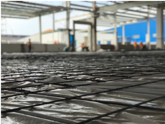
Fig. 5 M2 Global Pharmacy-cement curing
