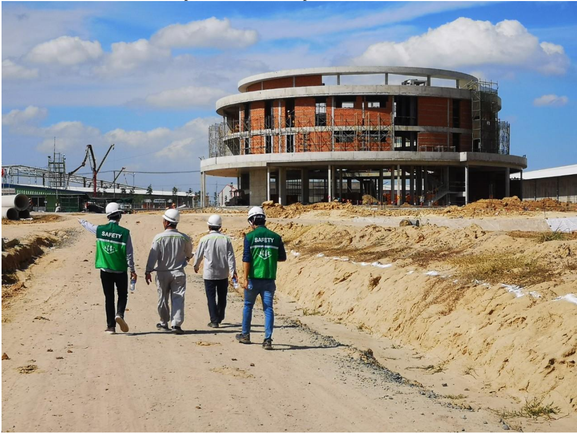
Figure 1: At the under-construction Headquarter of SAITEX Project
