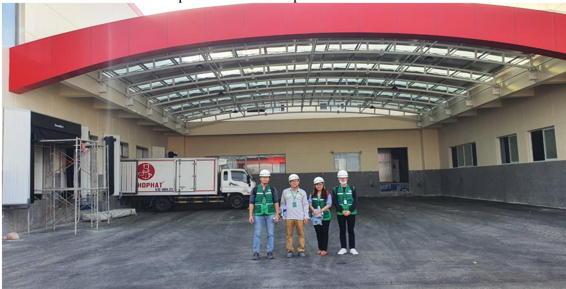
Figure 1: At the main entrance of Tho Phat Project
