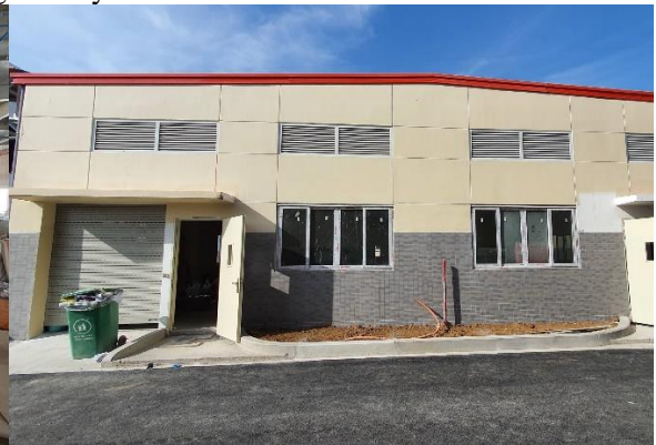
Front view of maintenance area
